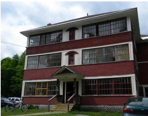
23: Saranac Cottage with Multiple Cure Porches (Photos by Paige Doerner)
